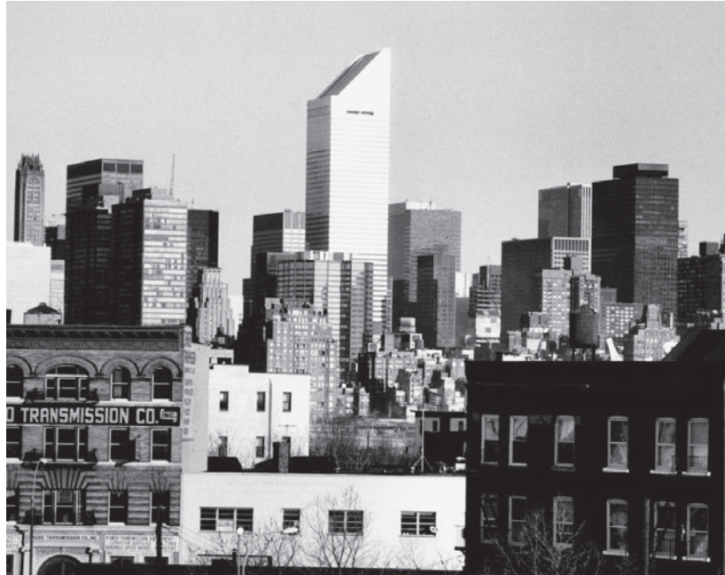
The Citicorp Center in Manhattan (white building, center top). Structural problems in the design of this building led to a retrofit to ensure that the building could withstand extremely high winds. Photo by Marc Anderson, Simon & Schuster/PH College.
